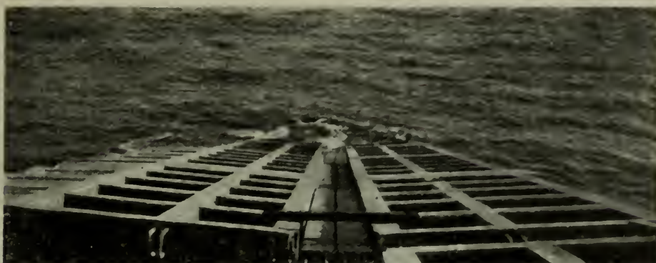
LOOKING SEAWARDS ALONG THE KEELWAY.
